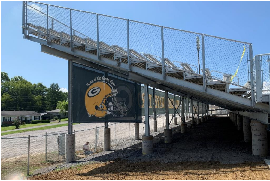
New Visitor side galvanized steel bleachers on sonotube foundations.
