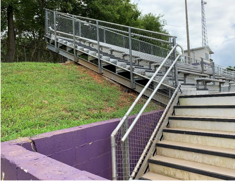
Side view of Visitor side galvanized steel bleachers built into the hill.
