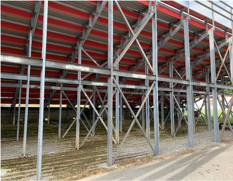
Back side of Home side bleachers with buried base plates.
